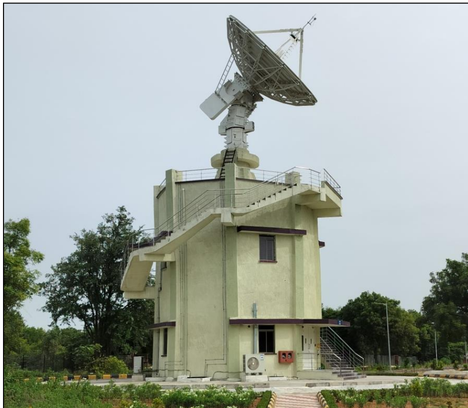
Tri-axis Antenna System Pedestal picture
