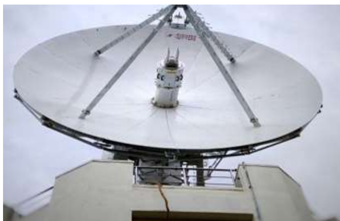
Figure 2 Dual band Feed installed in 7.5m Antenna System
